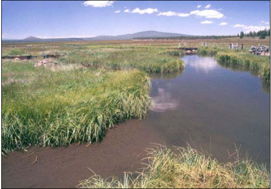
Photo 11-9. Klamath Marsh Refuge Rock Island Diversion Structure
