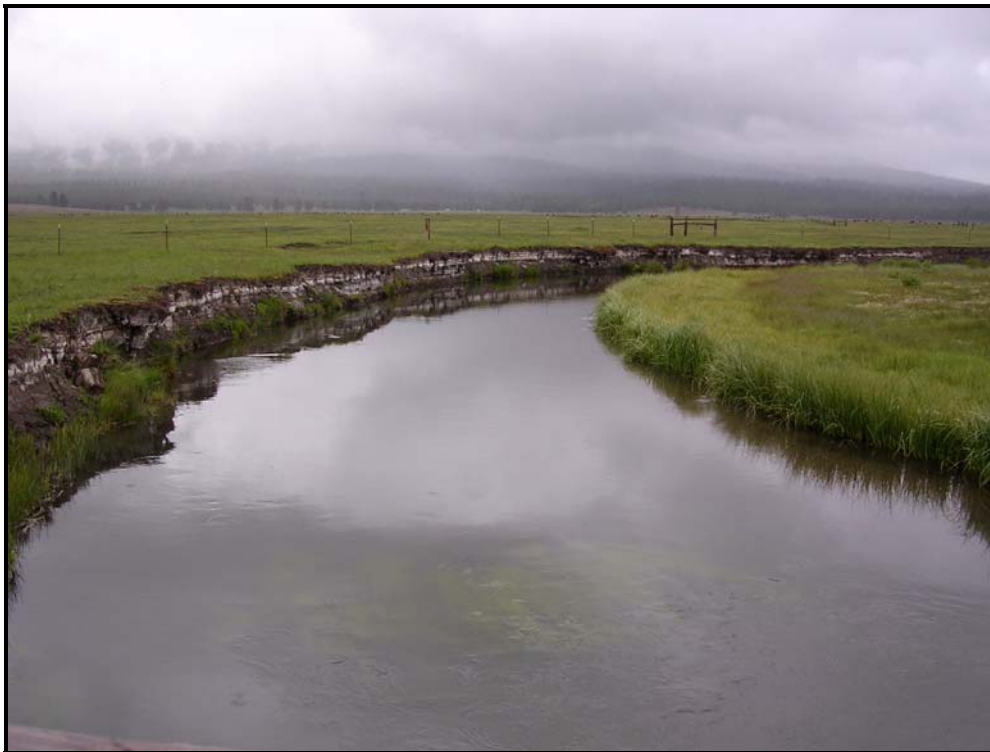
Photo 8-5. View of Incised Channel and Outside Bend Bank Erosion Downstream of Rocky Ford
