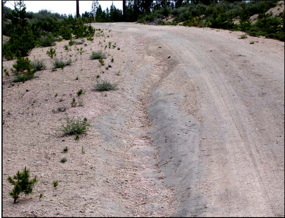
Photo 8-2. Gully along Steep Section of Road that Contributes Directly to Stream Channel
